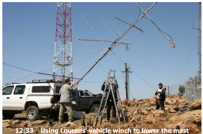
12:33 Using Lourens' vehicle winch to lower the mast
