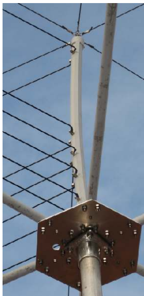
Nylon crimped to reflector
